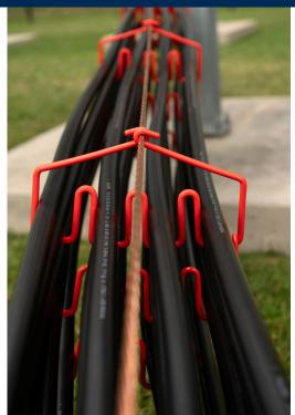
ModulAir™ can be used with the CAB® Solar patented integrated grounding system.
