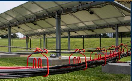
CAB Solar Cable Management products are ideal for tracker, ballasted or fixed installations. CAB multi-carrier hangers safely separate bundles of cables to meet NEC requirements. Numerous standard designs are offered to safely support large bundles of string wires, DC feeders, as well as AC, data or other cabling. Custom hanger configurations are available to meet specific project requirements.
